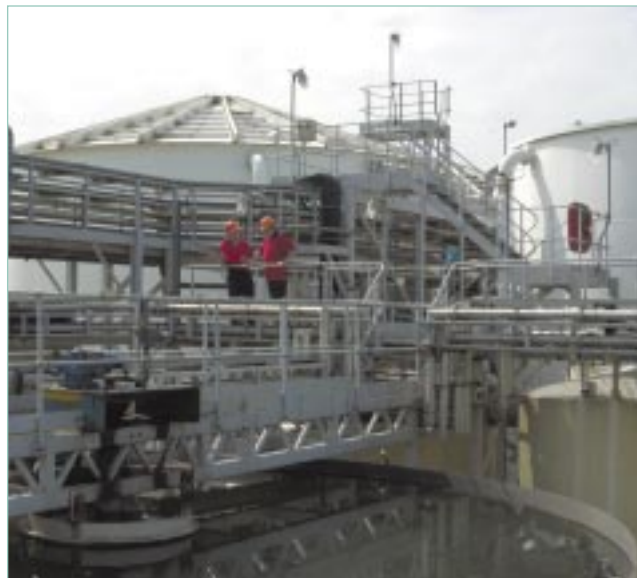
Checking the waste water treatment plant efficiency
